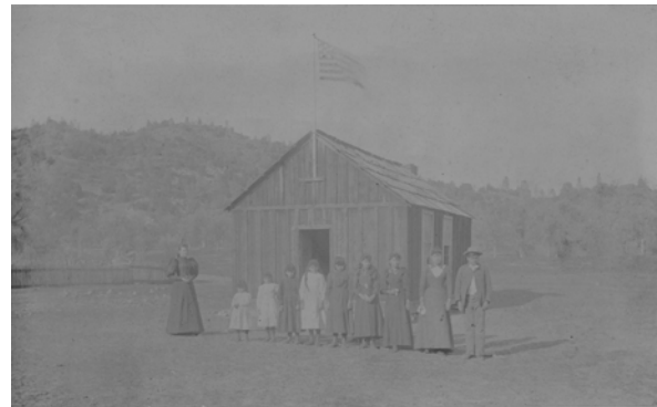
Poso Flats School Glennville, California
