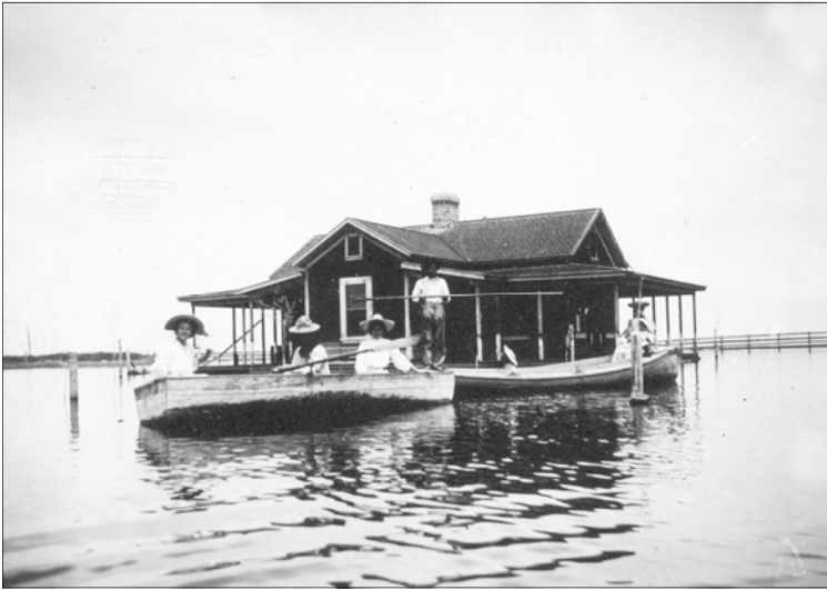
Flood waters surround the Lakeside Ranch Headquarters after the levee broke.
